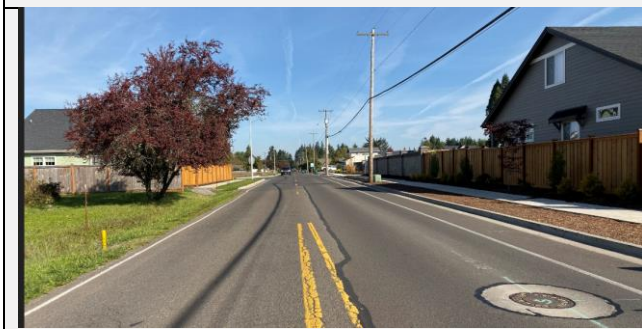
Incomplete Sidewalks Between Ayres Rd. and Ashbury Dr.
